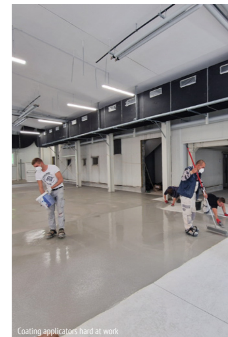
Coating applicators hard at work
