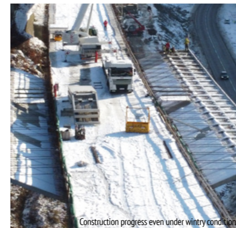
Construction progress even under wintry conditions
