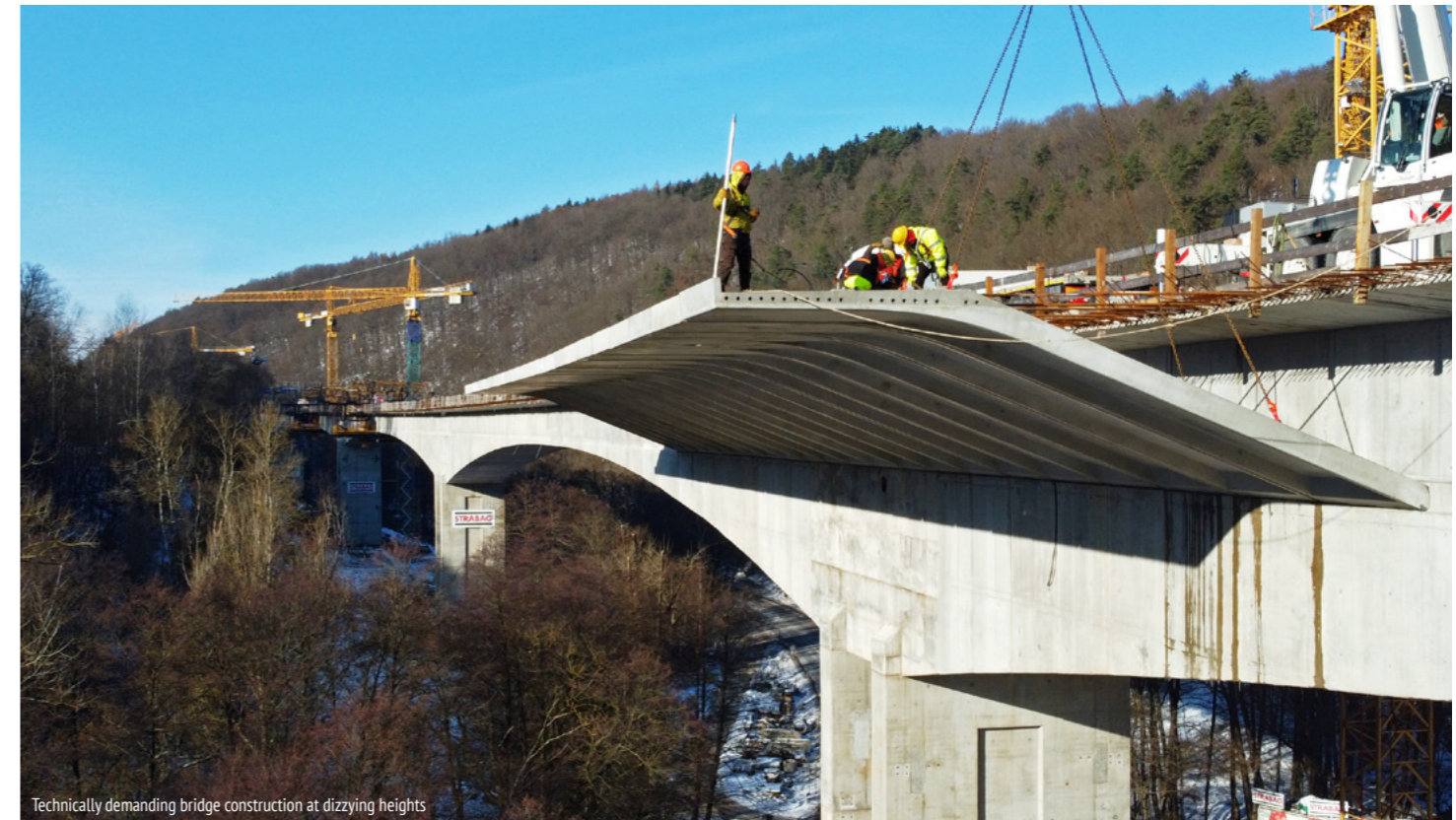
Technically demanding bridge construction at dizzying heights
