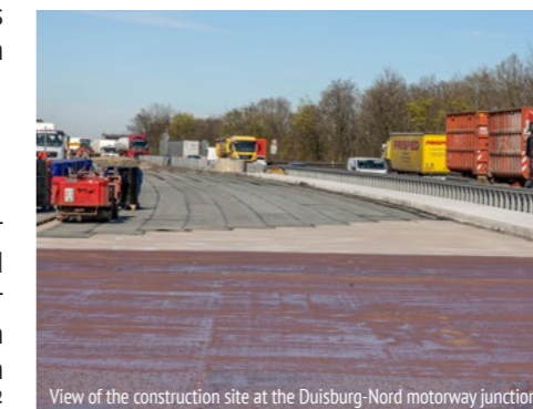
View of the construction site at the Duisburg-Nord motorway junction
