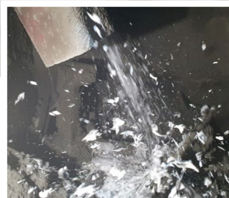
The foam produced with the MC-AirTec generator features highly stable micro-air voids which are introduced prior to injection into the premixed concrete.
