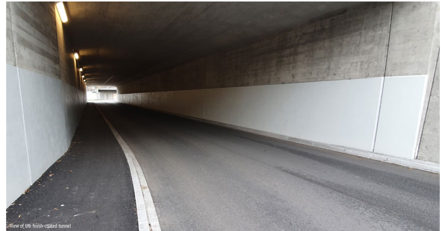
View of the finish-coated tunnel
