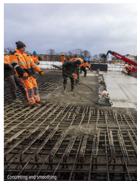
Concreting and smoothing
