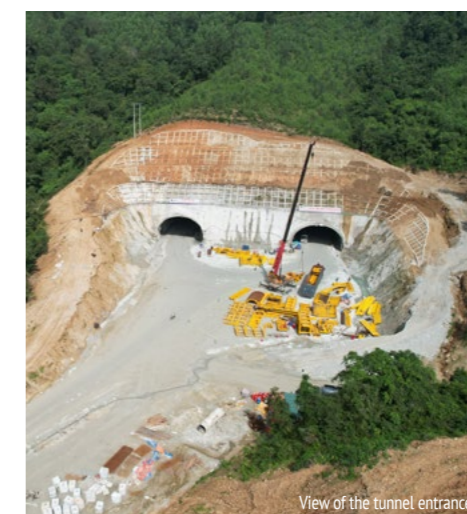
View of the tunnel entrances
